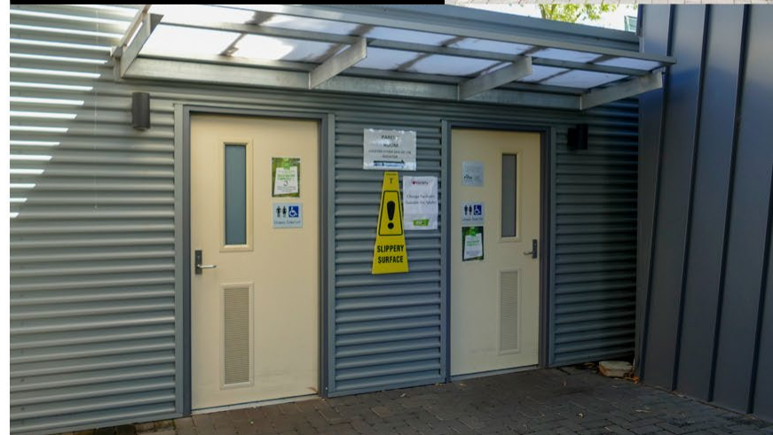
Toilets next to Wisteria Café
